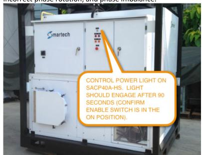
Please take note that the POWER CONTROL panel of the SACP rental units should only be opened and reviewed by a licensed electrician and/or a factory authorized service representative. Electric shock and bodily harm can result from contact with any power components.
