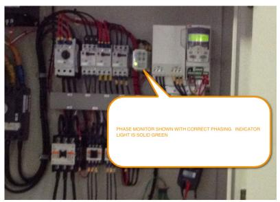
After 90 seconds the control power light should be powered (on the outside of the control panel) if the ENABLE SWITCH is in the ON POSITION. If the control power light does not come on after 90 seconds it it recommended to check the status of under voltage, over voltage, incorrect phase rotation, and phase imbalance.
