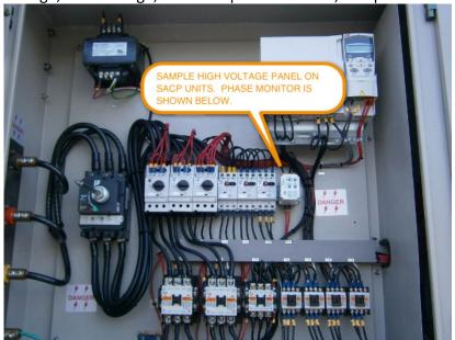
When a SACP rental unit is provided with clean power (with correct phasing) the phase monitor relay indicator light should be in a SOLID GREEN state.
